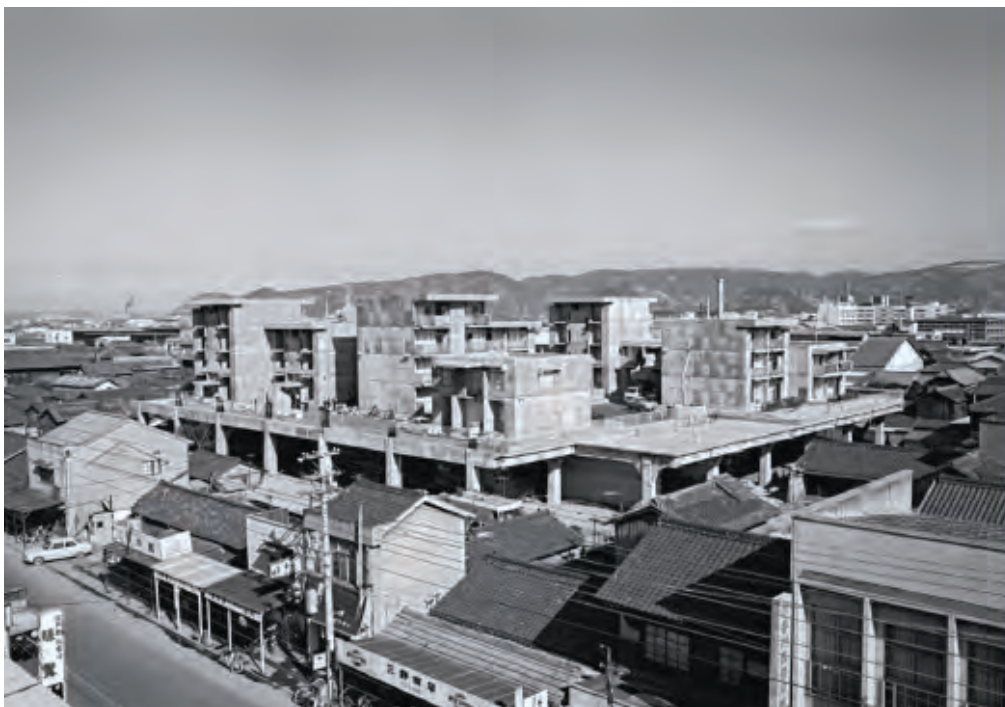
(above) Sakaide from south east, c. 1968 Image Credit: Osamu Murai 13
